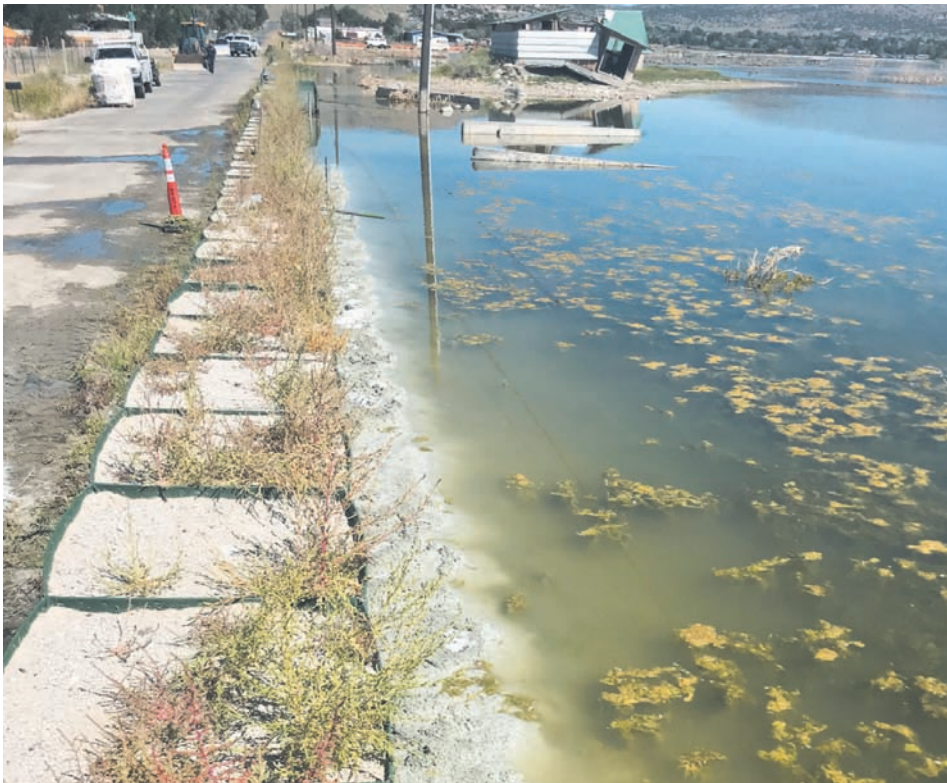
A HESCO barrier after bentonite was applied to it.
